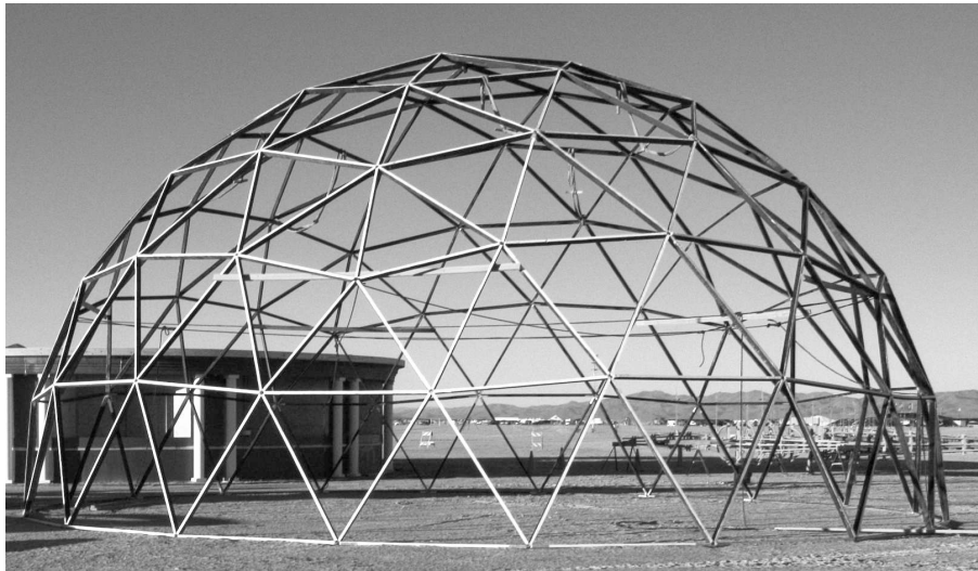
Figure 12: 4V Dome at Burning Man 2004
